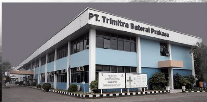
TRIMITRA plant, JAKARTA, INDONESIA
